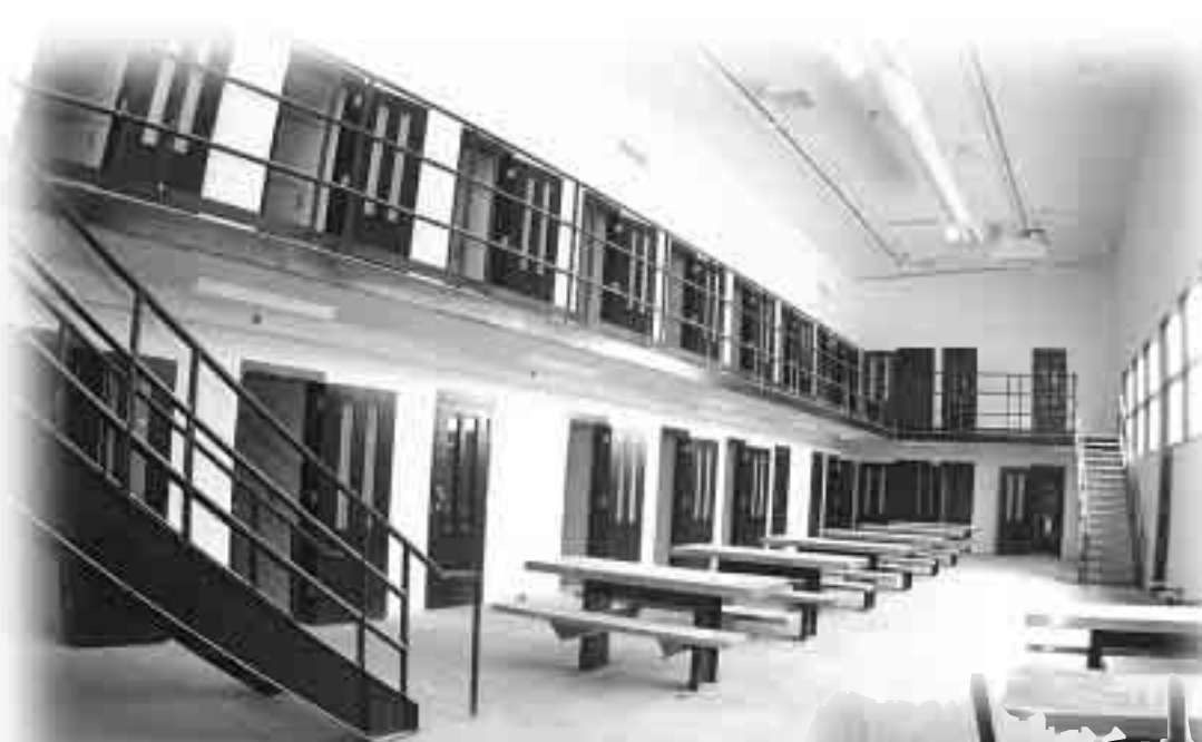
Left, natural light can be seen shining in from the right side of this completed prison cell block within the 432-bed new Lea County Detention Facility in Lovington.
